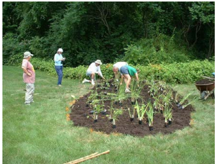
Volunteers working on the construction of a raingarden
